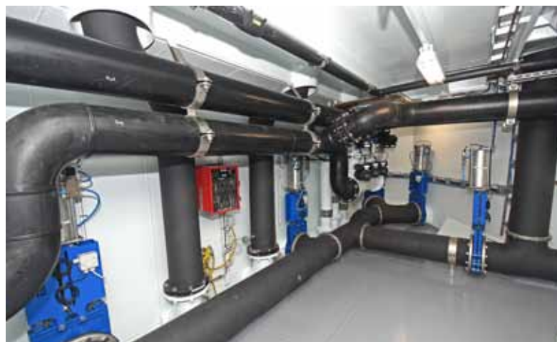
▲ The lower RSW manifold room.
