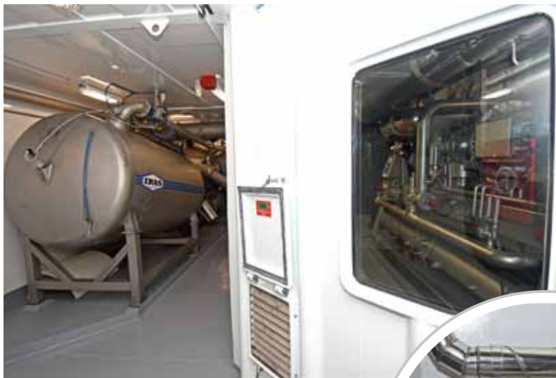
▲ A window enables quick visual checking of the refrigeration plant on the shelterdeck.
